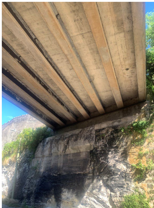
Photograph 12 – Overview of the bridge deck soffit
