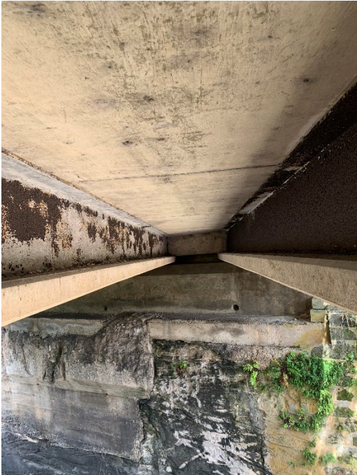
Photograph 13 – Bridge deck soffit
