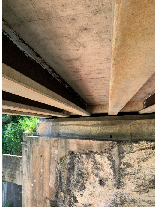
Photograph 5 – Example of prestressed concrete encasement in good condition
