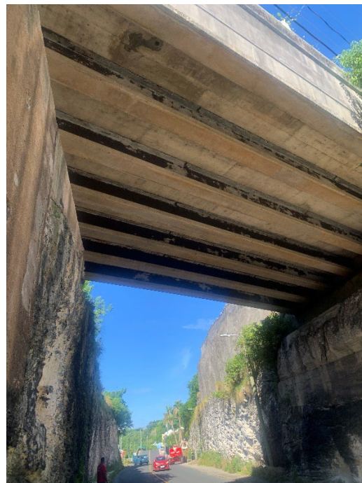
Photograph 6 – Example of prestressed concrete encasement in good condition
