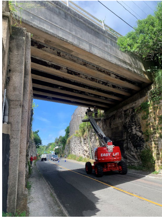
Photograph 1 – Access to the overpass was via a MEWP
