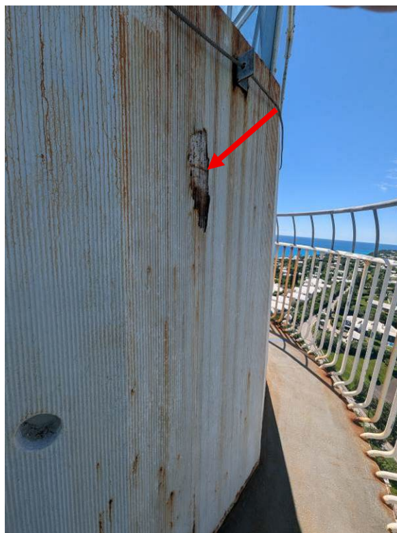
Photograph 30: Upper gallery section of northern façade
