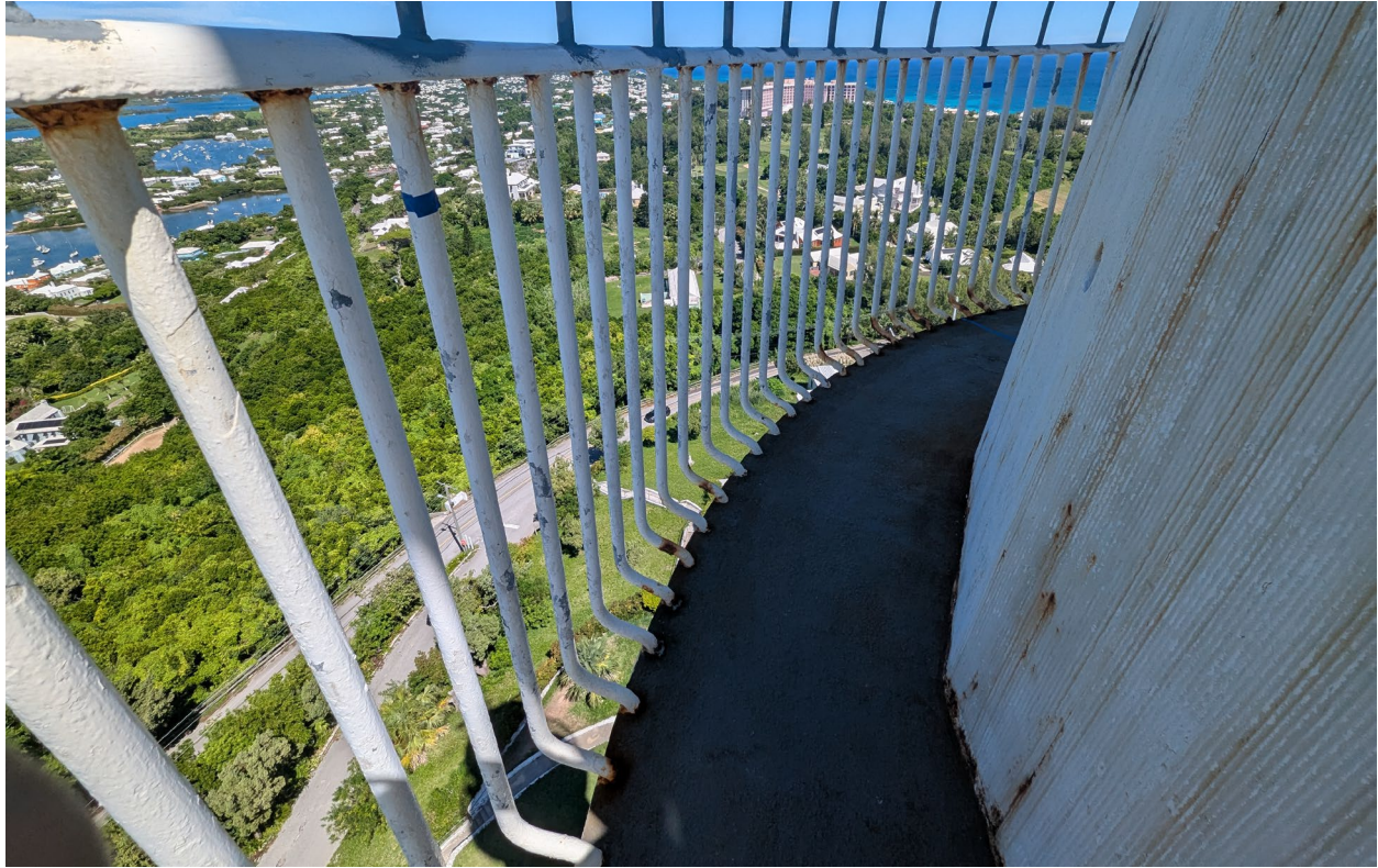
Photograph 11: Lower gallery railings in Section 3 (Bars 041-060)
