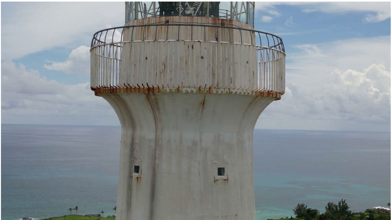
Photograph 2: Northern elevation of gallery platform
