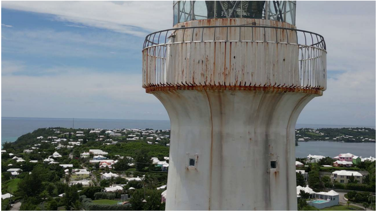
Photograph 3: Eastern elevation of gallery platform
