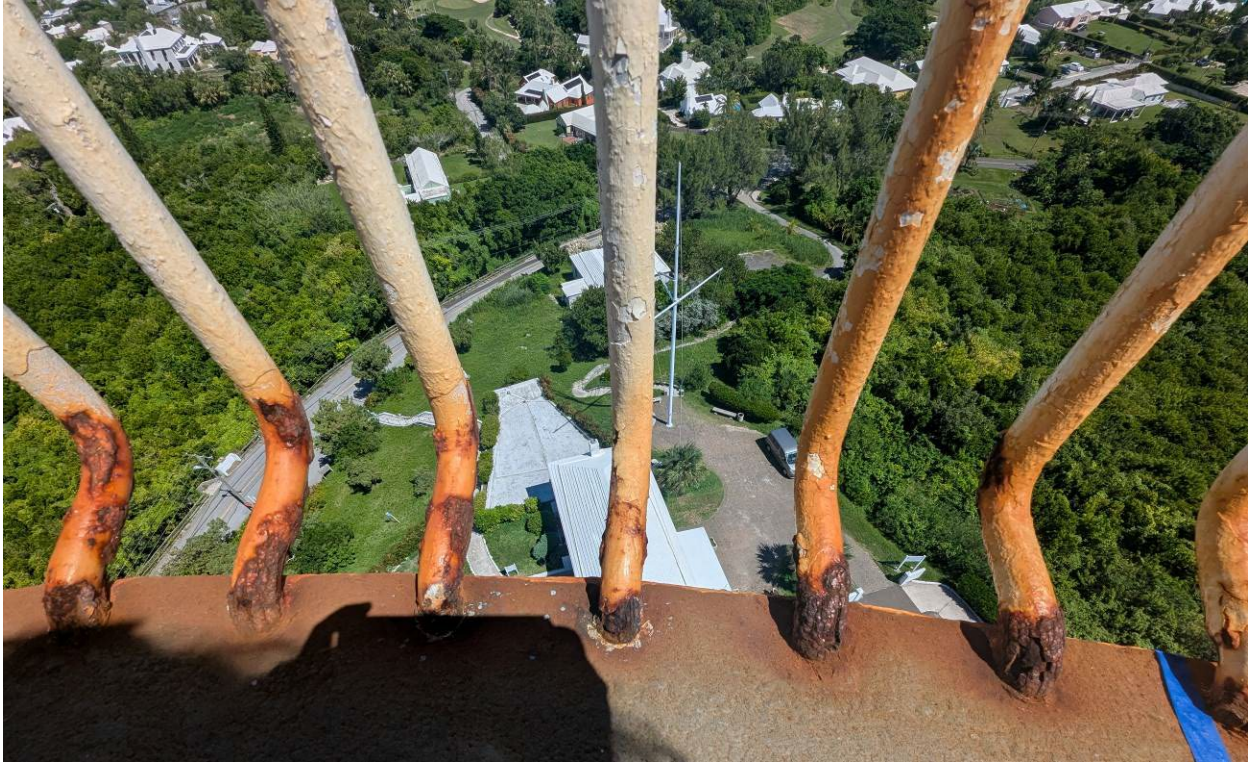
Photograph 9: Lower railings connection to platform in Section 2 (Bars 021 to 026)
