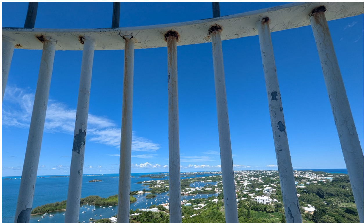
Photograph 12: Typical lower railings connection to intermediate rail in Section 3
