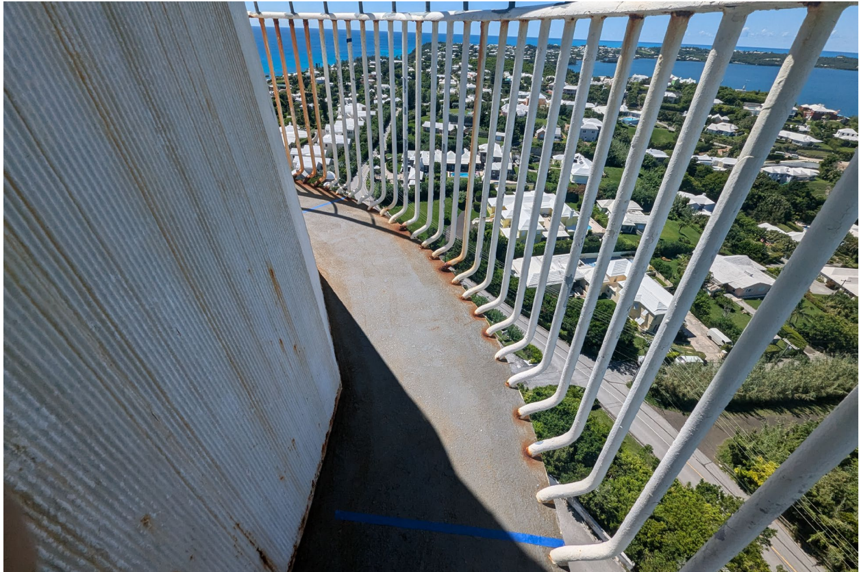
Photograph 13: Lower gallery railings in Section 4 (Bars 061-080)
