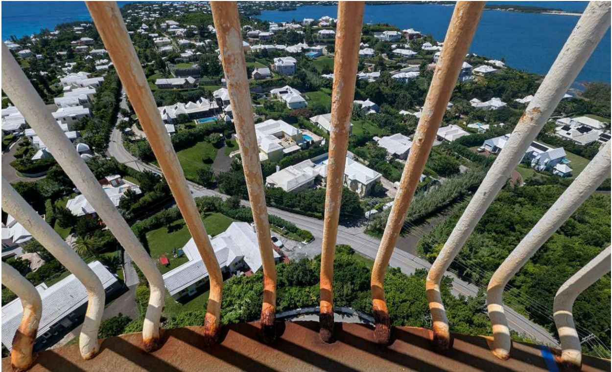
Photograph 17: Lower railings connection to platform in Section 5 (Bars 081-089)
