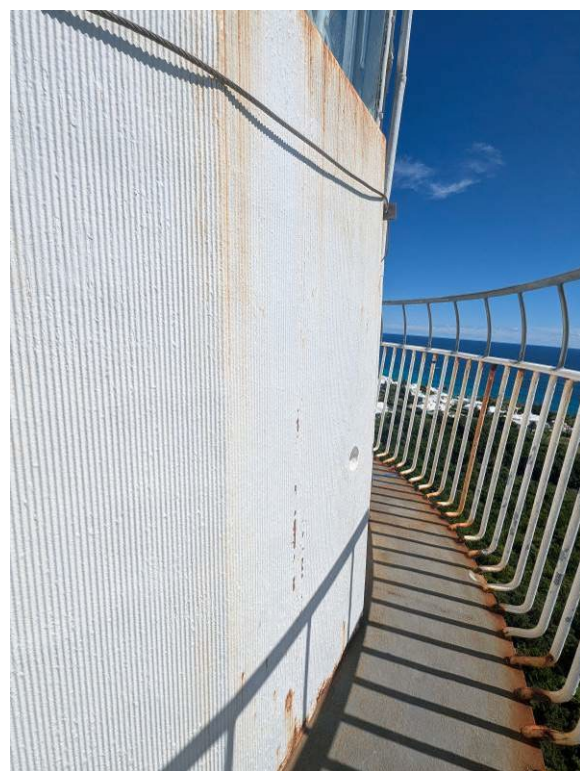
Photograph 31: Upper gallery western façade
