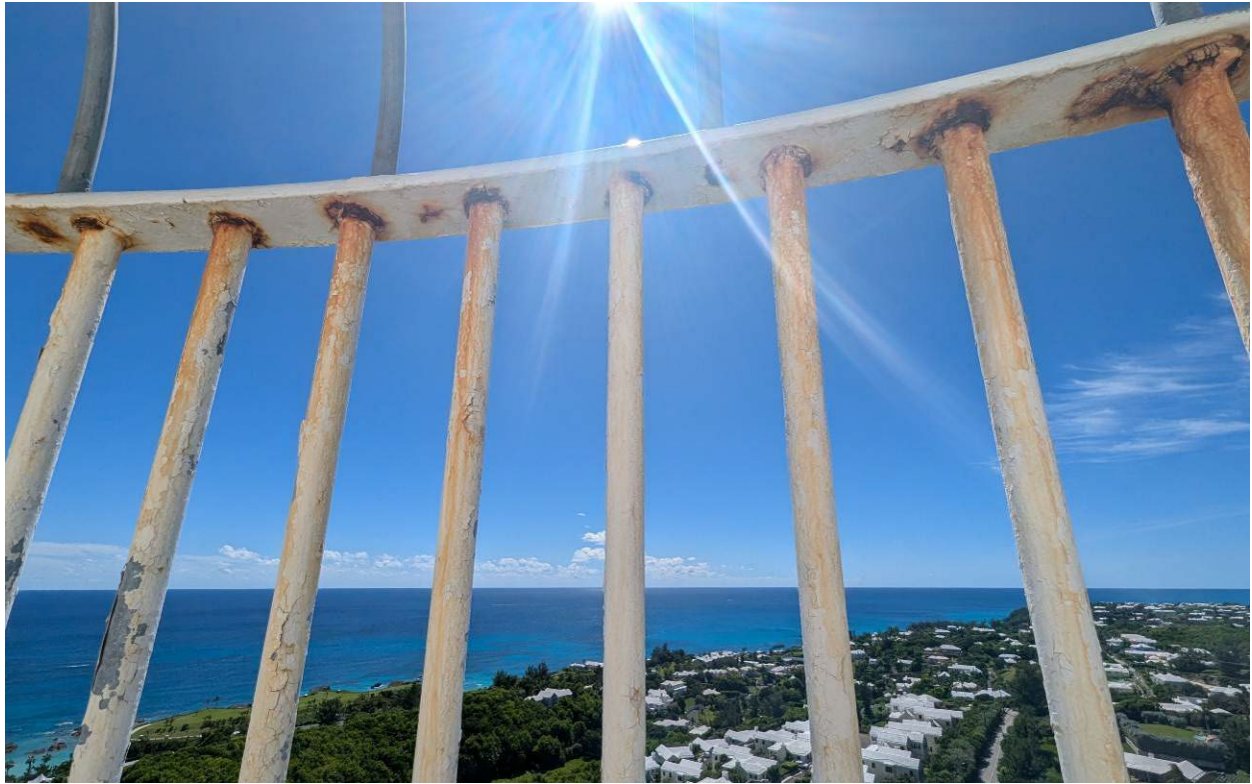
Photograph 22: Lower railings connection to intermediate railing in Section 6 (Bars 101-106)
