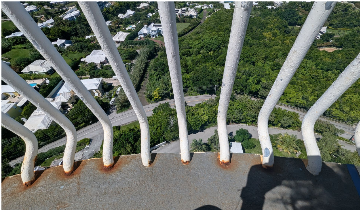
Photograph 14: Lower railings connection to platform in Section 4 (Bars 061-068)
