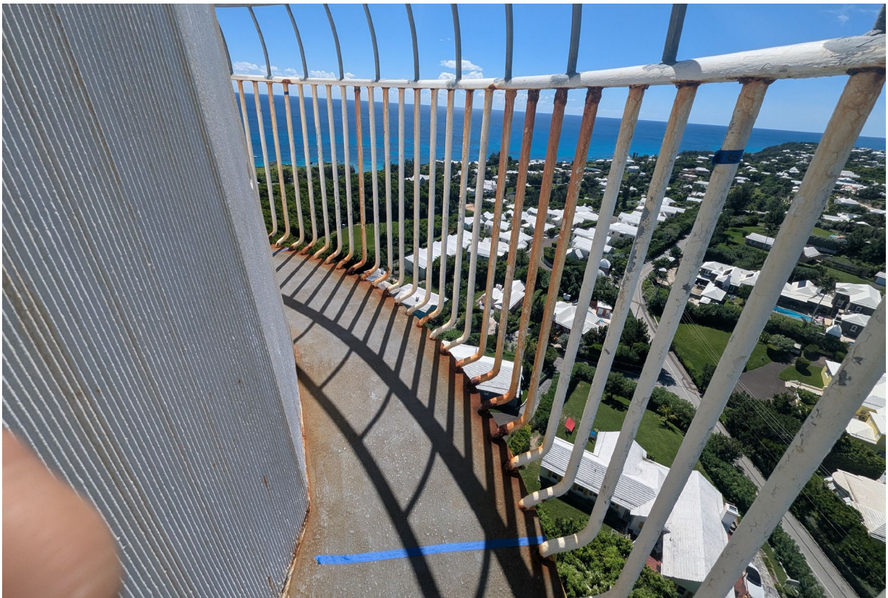
Photograph 16: Lower gallery railings in Section 5 (Bars 081-100)
