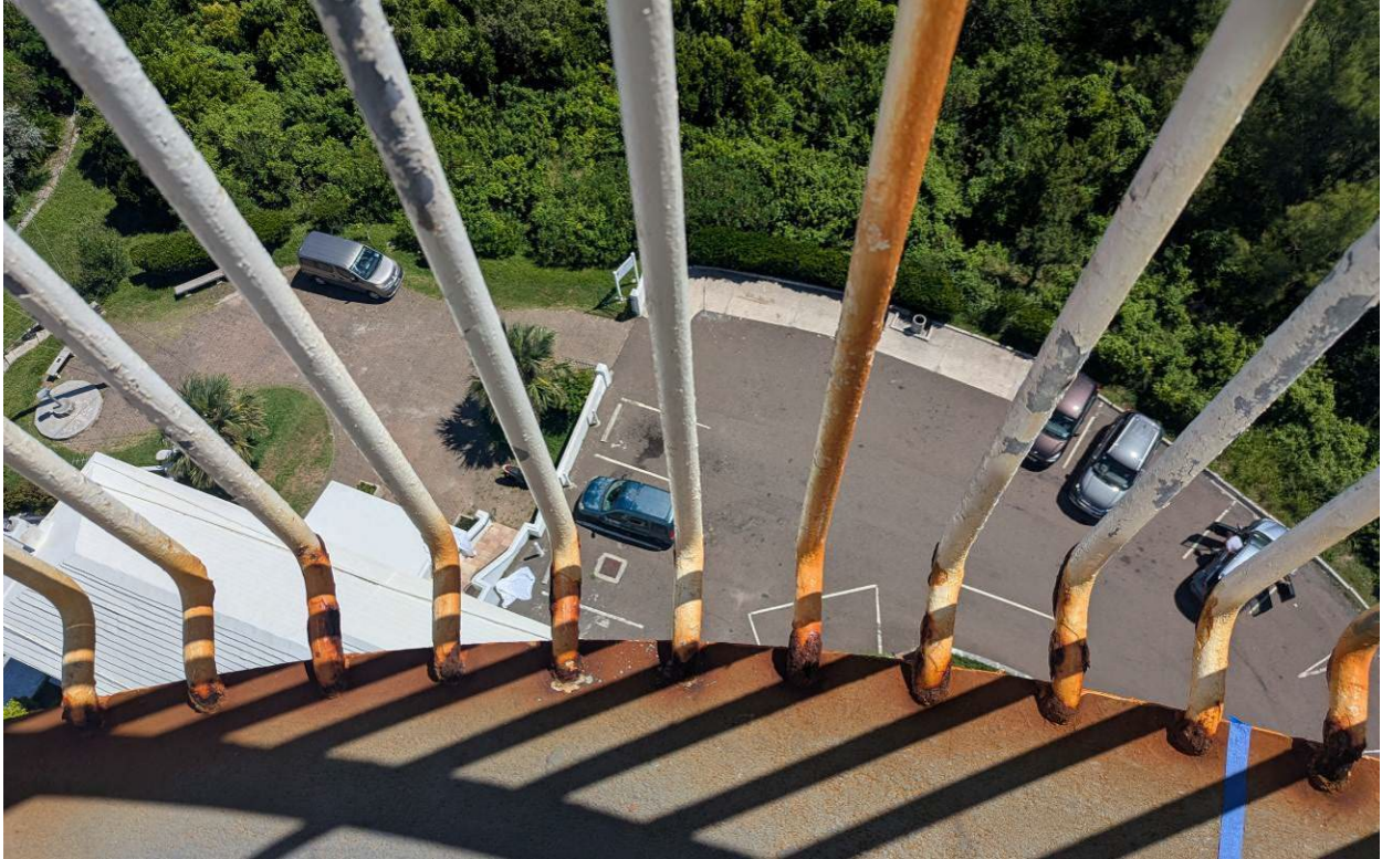
Photograph 5: Lower railings base in Section 1
