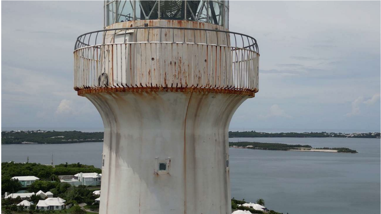
Photograph 1: Southern elevation of gallery platform
