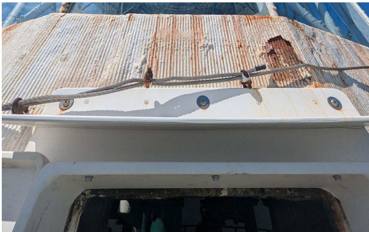
Photograph 28: Upper gallery southern façade (above doorway)
