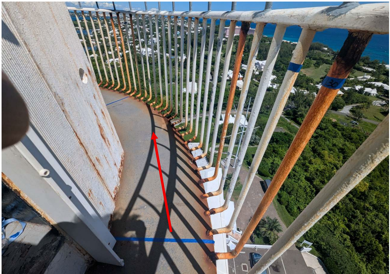
Photograph 4: Lower railings Section 1 (Bars 001 to 020) commencing from platform entry door
